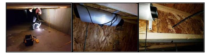
A single UVAIRx Ux105 unit was securely fastened with tamper-resistant fixtures in each of the crawlspaces at the treated construction sites and power was supplied from the temporary construction power meters present at each site. Each site was inspected on at least a weekly basis to ensure that the units were properly functioning.
